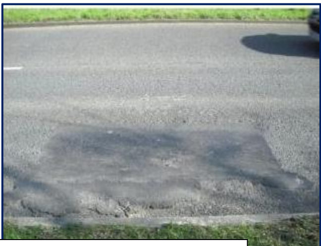
“Market Leading” permanent solvent-based cold surfacing material – catastrophic failure after a 12 month period.
