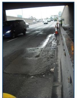
underpass/A13) in an area with a high water table. This allows the water to come up through the material and drain away, also used in the Dartford tunnel for pothole repair. This patch of Viafix OPA was added Nov 2011 and is still in place, other hot laid patches were only staying in place for roughly six weeks, due to pressure building up below the surface.
