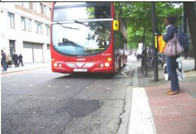
Open to traffic immediately
