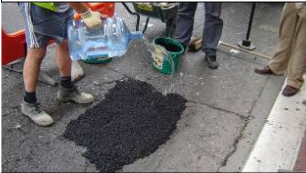
Add water in dry conditions to start the curing process
