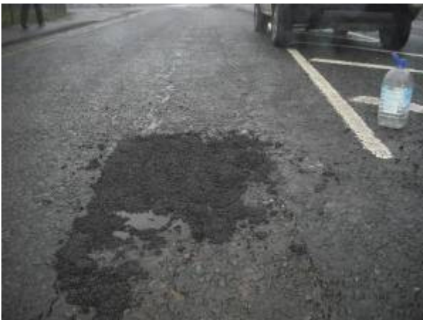
A permanent repair in freezing, wet conditions, without cutting or TM is possible with Viafix – Repair took 30 seconds
