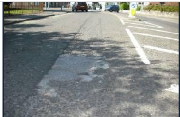
After Viatec was laid in foul weather, freezing conditions and trafficked immediately, it still stands in the road 22 months later (Aug 2012)
