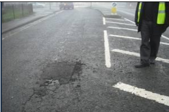
After Viatec was laid in foul weather, freezing conditions and trafficked immediately, it still stands in the road 22 months later (Aug 2012)
